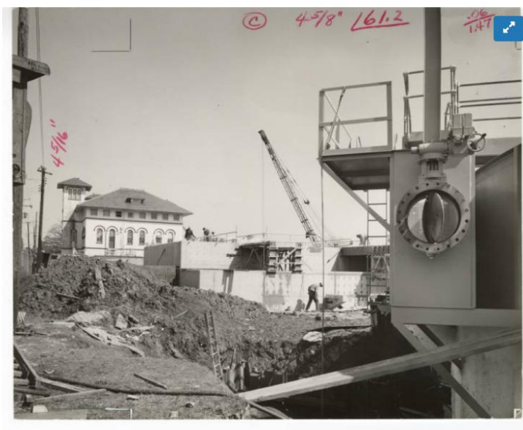
Figura 10. Algiers Water Purification Plant.
